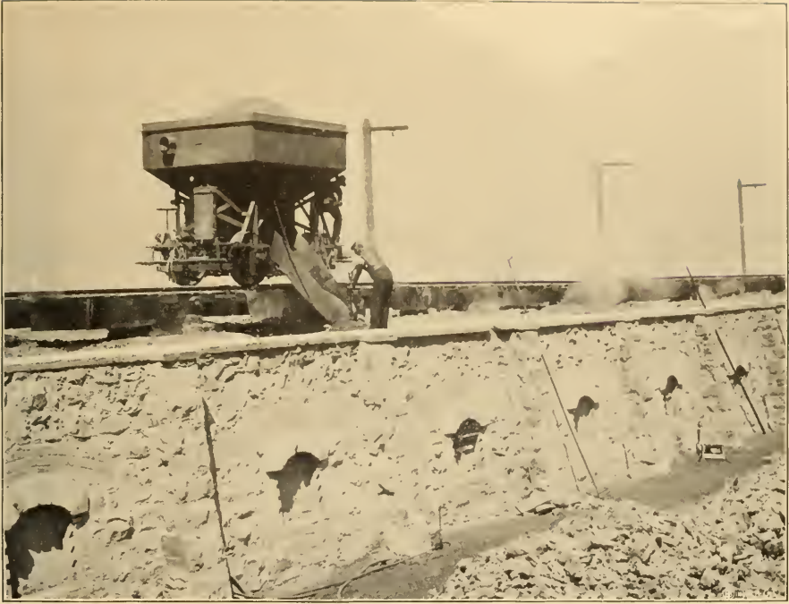
ELECTRIC TROLLEY—CHARGING COKE OVENS—FERNIE.
